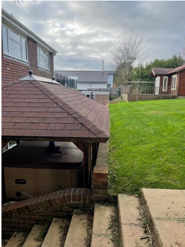
View looking west towards No. 35A
