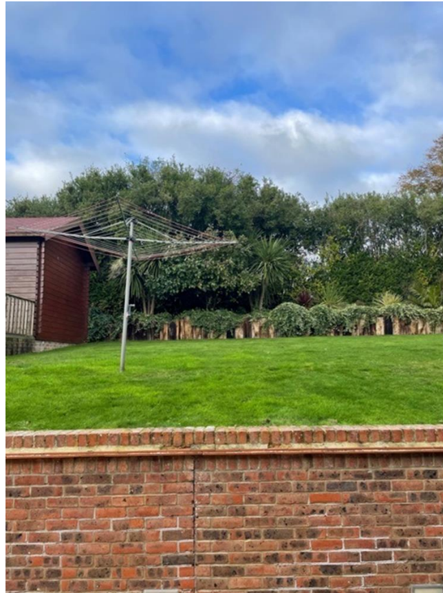
View looking towards the north (rear)
